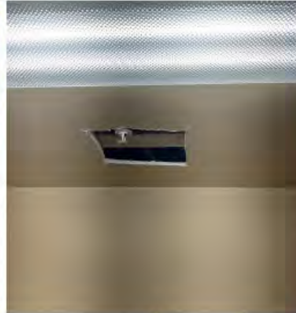
00296 - Restrooms - Bathtub/Shower (Common Area) - Apr 24 2025 11:35AM - K Fuqua CAPTION: Large hole around sprinkler head (1st floor hall)
